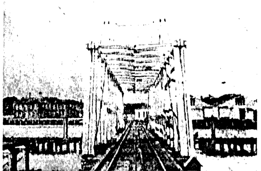
Fig. 52: Railroad bridge at Main St., about 1900
